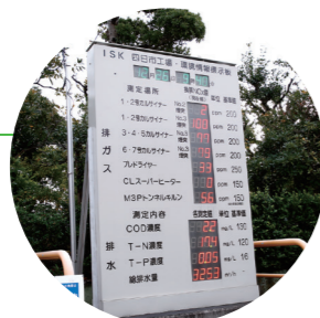
We release NOx concentrations in exhaust gas and other figures subject to water quality regulations.
