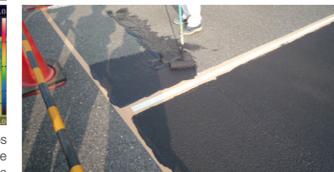
Applying black heat-shielding coating
