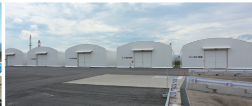
2023 Land leveling work is completed
