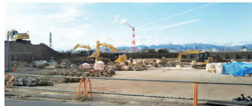
2018 Removal work is underway
