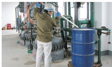
On-site guidance at the manufacturing contractor
